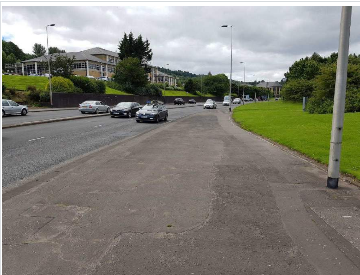
Figure 3.4: A8 (T) Footway
